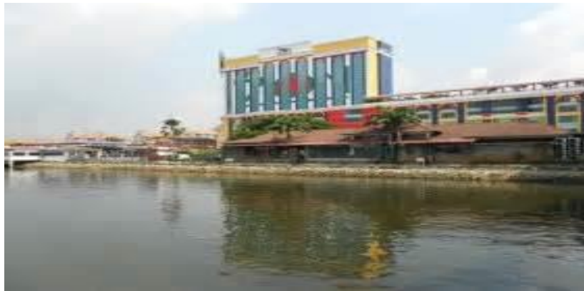
Figure 3: Port of Stulang Laut, Johor, Malaysia
