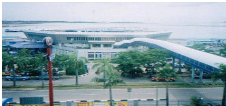
Figure 2: The bridge connecting between terminals and malls
